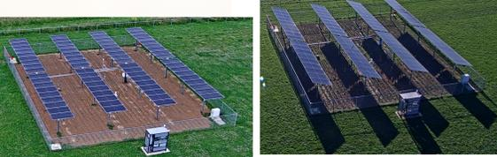
Figure 3 Photos of installation at two different periods of tracking: horizontal (left) and backtracking (right).
